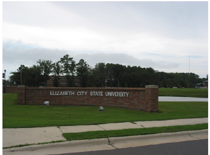
Fine Arts Entry: The campus wall alone is too low and lacks the necessary scale to define a true threshold. Supplementing the wall with plantings of differing scale and vertical architectural elements would help to visually mark the campus entry sequence.
