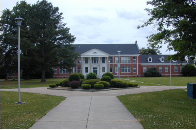
Williams Hall (1951), found on North Campus, is clad primarily in the typical campus red brick and uses precast accent bands to define a more pleasant scale and a white painted stucco to define the entry.
