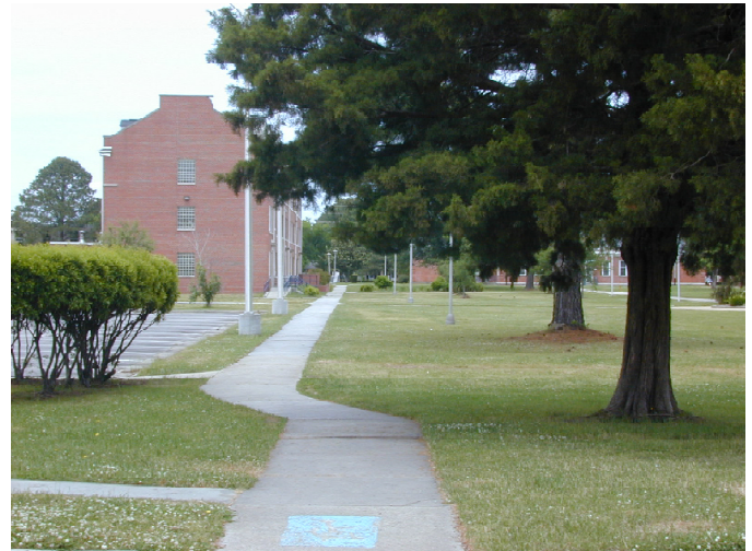
A missing edge on the western side of the North Campus Lawn allows one a clear view of the visually obtrusive perimeter parking lots.
