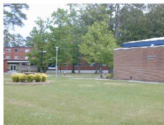
Under-scaled landscape treatment in front of Bedell Cafeteria.
